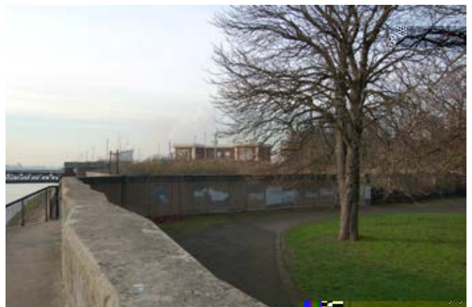
Figure 18. Walls at Royal Victoria Gardens
